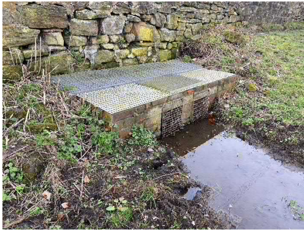
Photo 1: Culvert under Lamesley Road (TN2)
